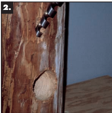
2. Drill a filling hole at a 45° angle
